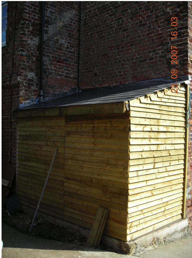
Extension at Pinbrook House, Chenyegate Lane
